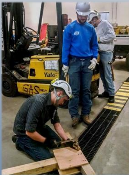
Assembly of shoring.
