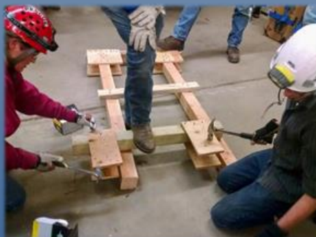
Nailing plates to Double-T shoring.
