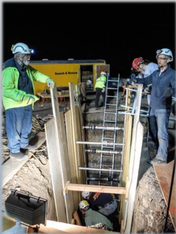
Trench rescue practical shoring system in place
