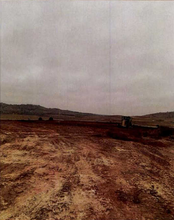
Existing dirt work and disturbance area.
