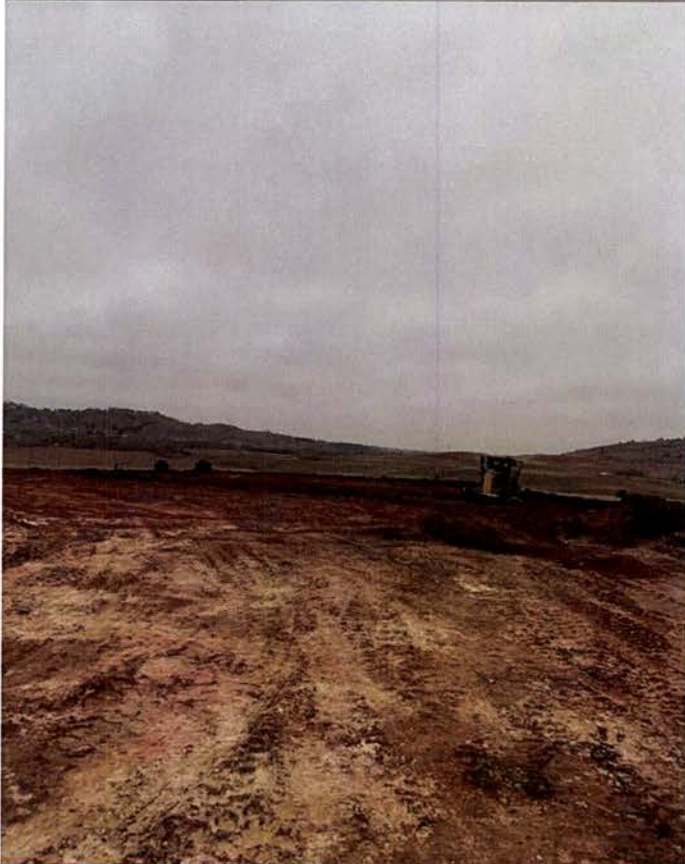
Existing dirtwork and disturbance area.
