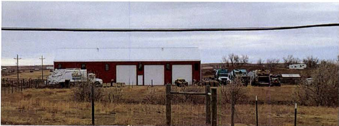
November 2019 - Subject Property showing proposed Contractor's Equipment Storage Yard.
