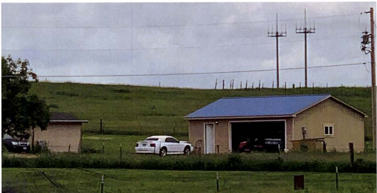
Distance of garage from existing shed (shed on or over property line of Lot 7)
