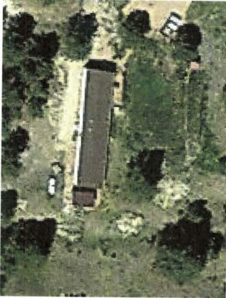
Former Single-wide Mobile Home (2017)
