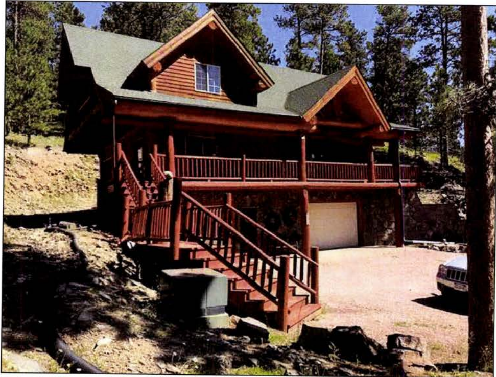
Site Visit, August 19, 2019.
