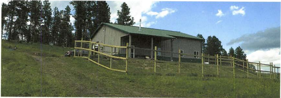
Existing pole barn with living quarters.
