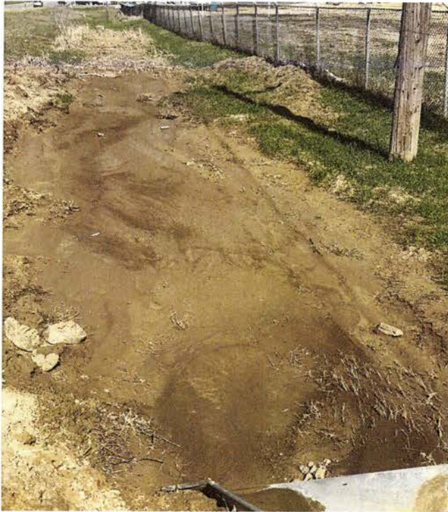
Sediment in road ditch on the south side of racetrack
