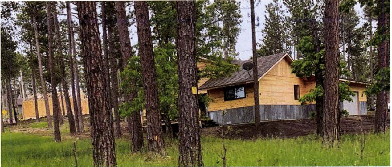
Guest house and single-family residence
