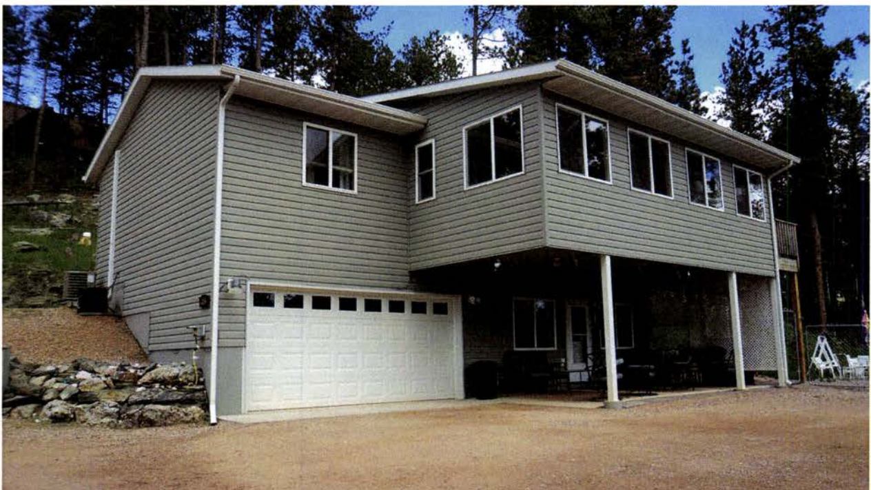
Site photo from 6/11/2019.
