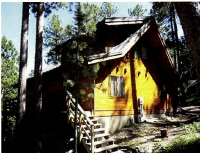
Site Visit June 6, 2019
