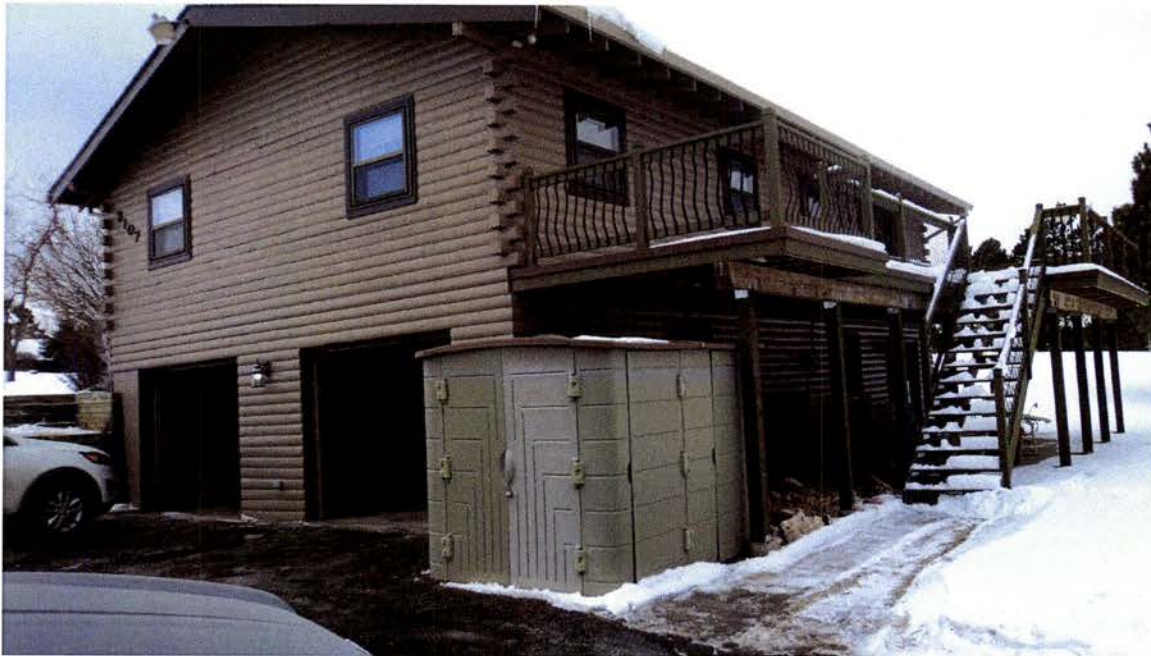
March 1, 2019 site photo.
