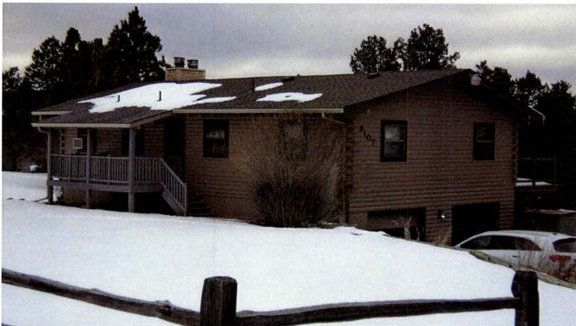
March 1, 2019 site photo.
