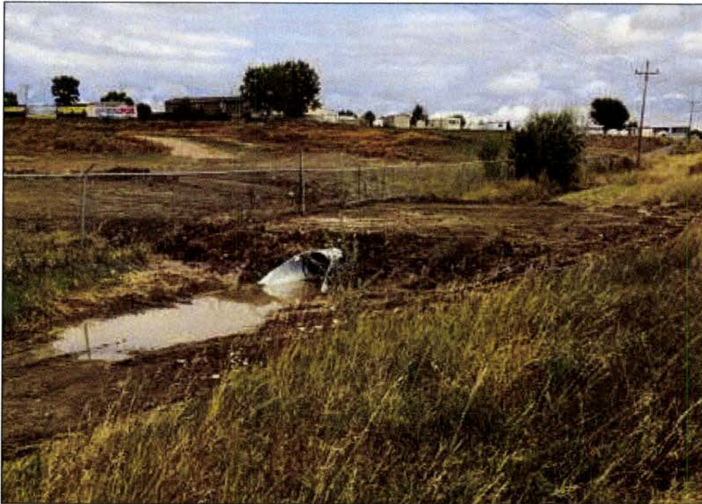
New approach off of E. Highway 44
