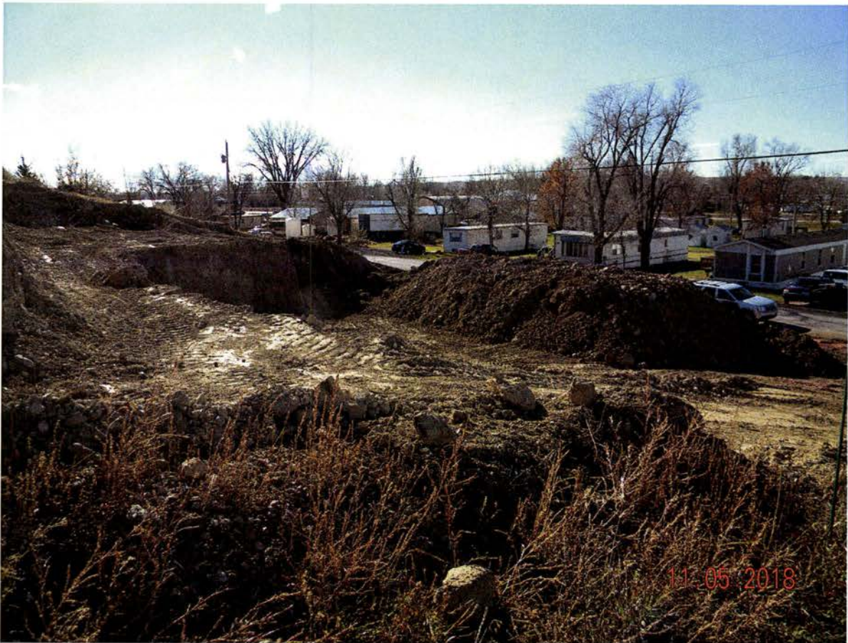
Foundation Excavation Area (11/5/18)
