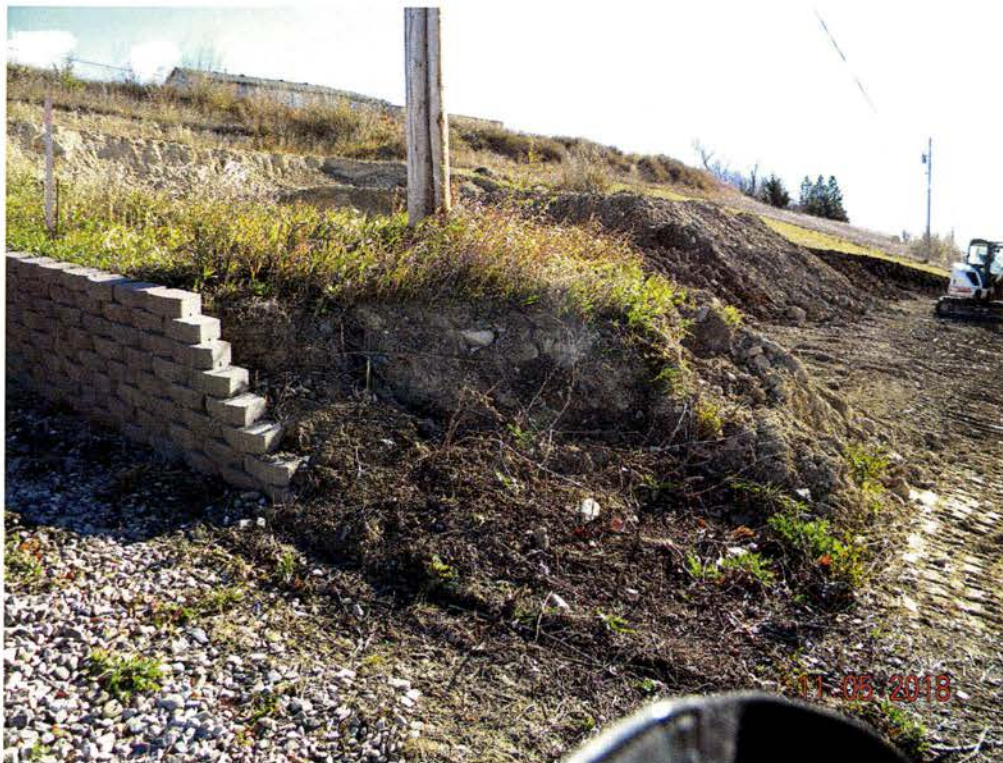
Retaining wall on property to the west (11/5/18)
