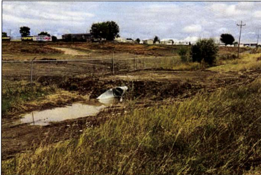
New approach off of E. Highway 44
