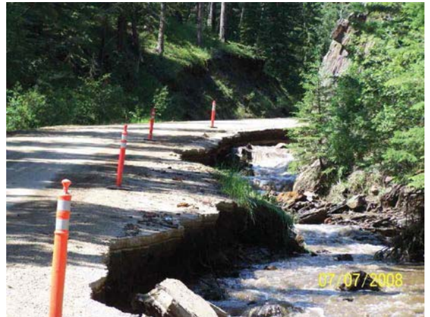
Photo 1. Example of Erosion on South Rochford Road
