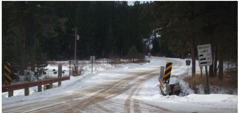
Photo 2. Weight limit restrictions on the Rapid Creek Bridge
