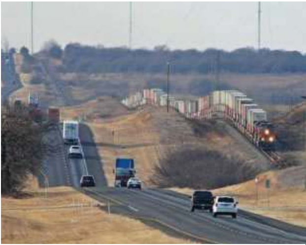
Photo 4. Example of a vertical curve in a roadway.
