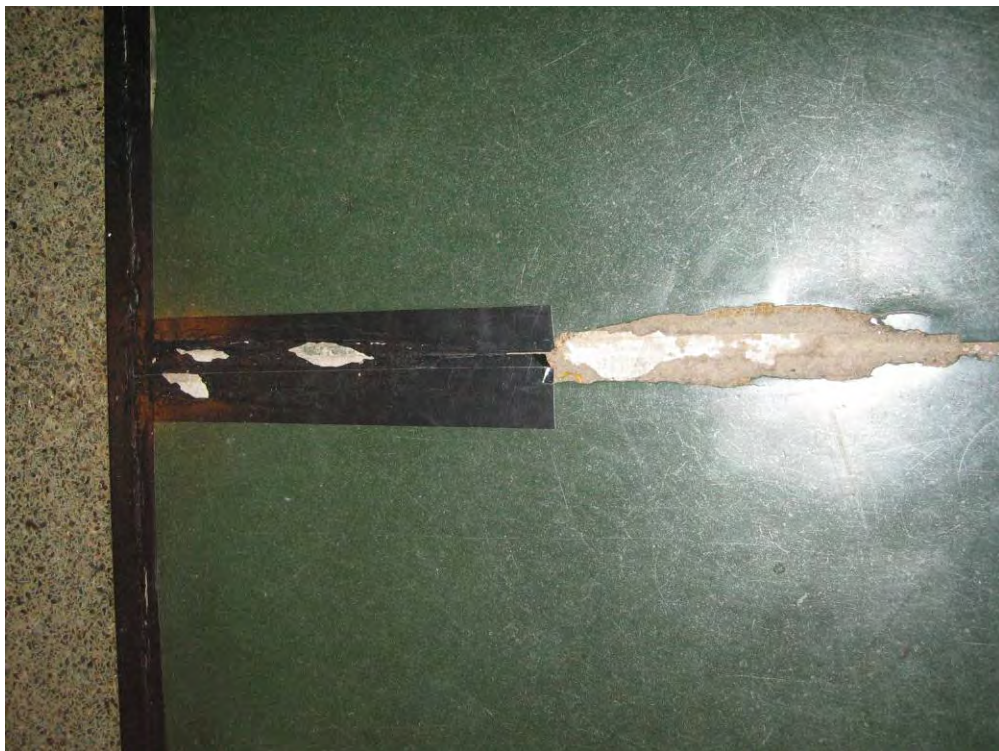
Cracked and peeling linoleum with tape
