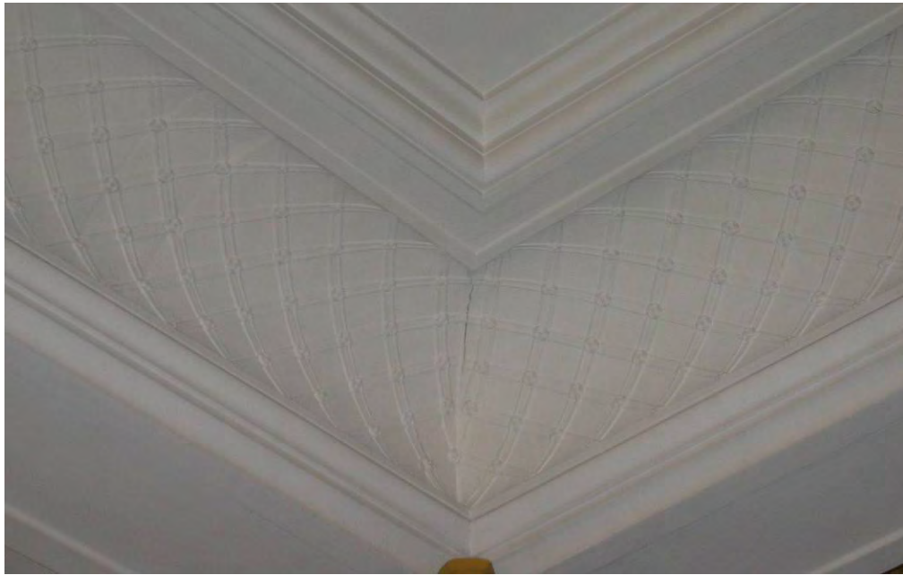
Crack in the corner of the covered edge of ceiling on second floor
