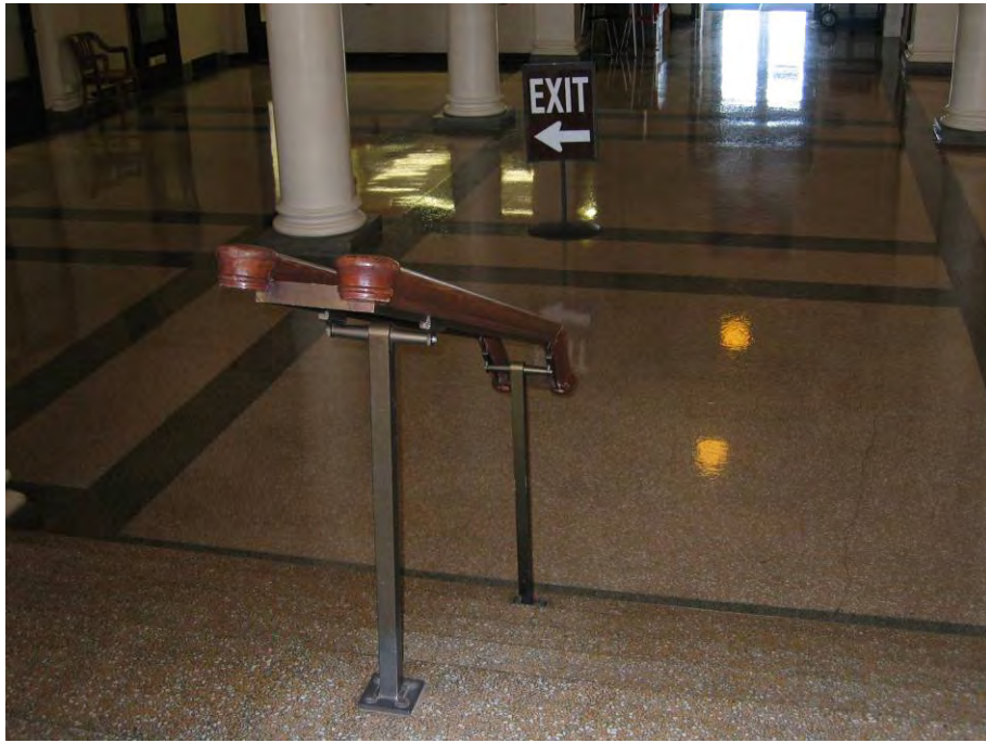
Terrazzo floor and steps from the foyer into the lobby
