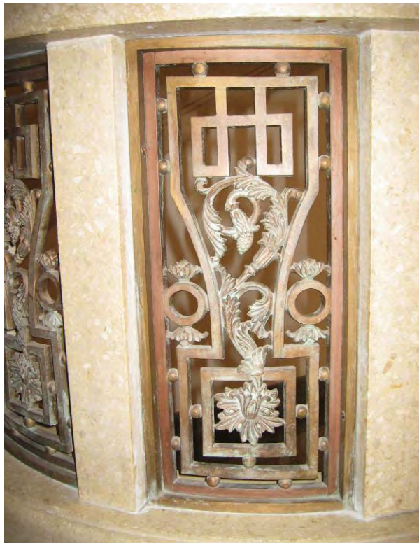
Close-up for bronze grillework in the marble staircase
