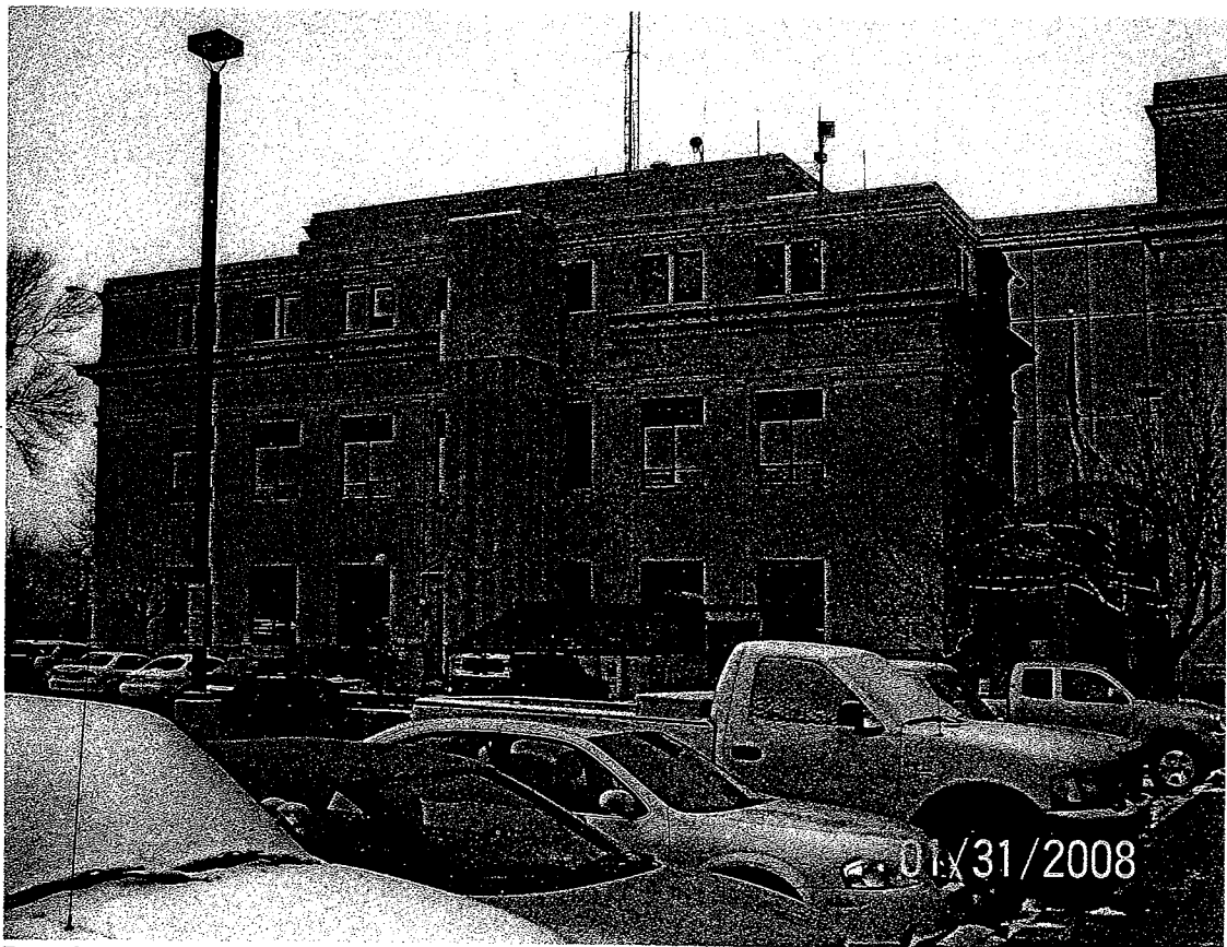
Pennington County Courthouse (South Façade)
