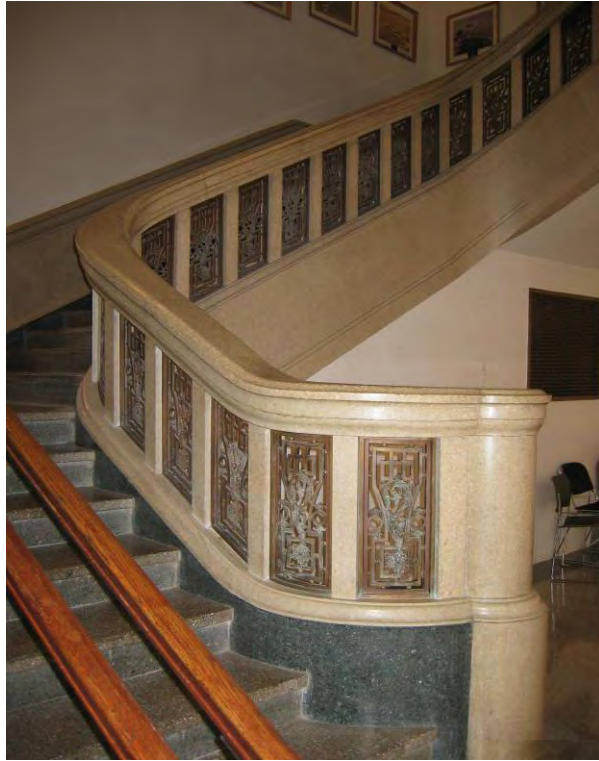
Stairs from first to second floor (east end of foyer)
