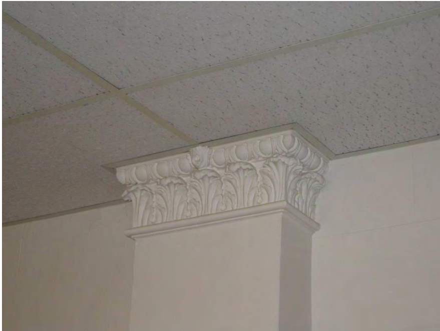
Drop ceiling cut into capital of pilaster in hallway
