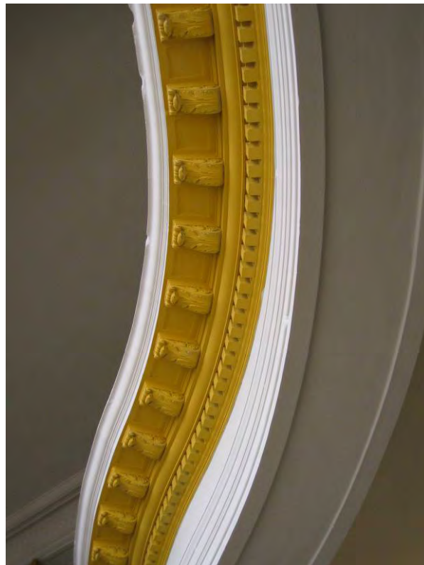
Cornice detail at balcony edge
