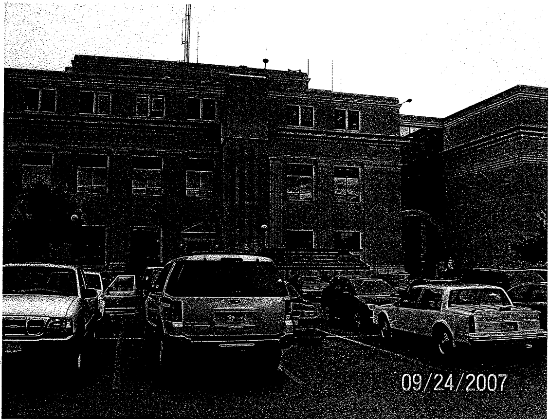
Pennington County Courthouse (South Façade)
