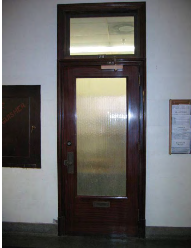
Original office door and transom located at west end of second floor
