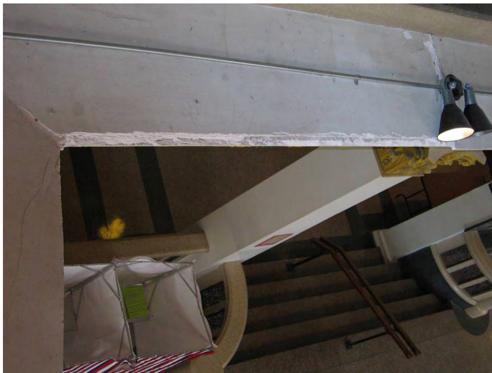
Top edge of cornice at balcony shows crumbling plaster
