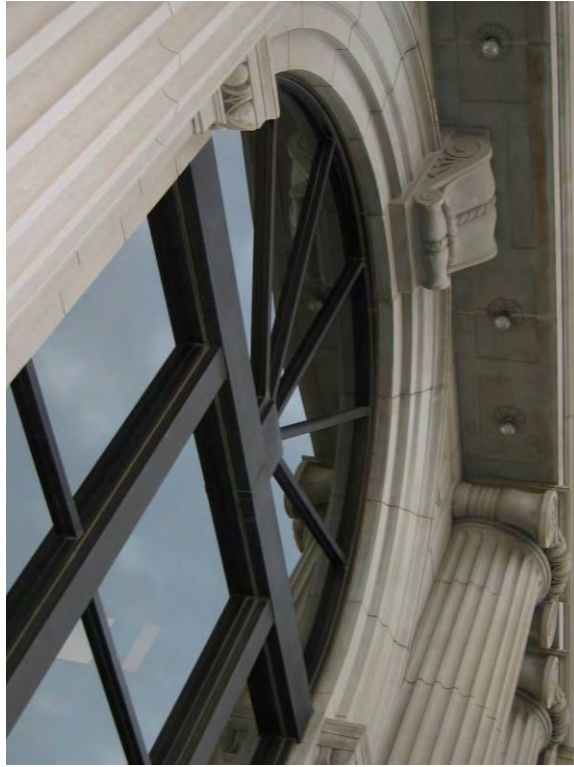
Detail of rounded arch window with keystone and egg-and-dart detail at the arch spring line
