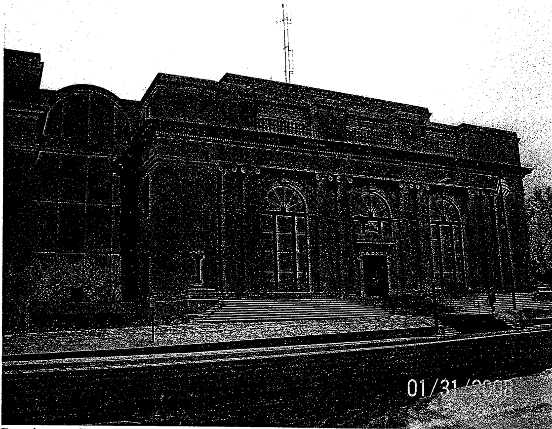
Pennington County Courthouse (North Façade)
