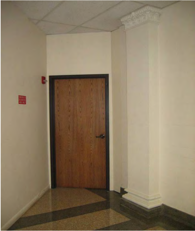
Wall and doorway addition which closed off the corridor on the north side of the courtrooms
