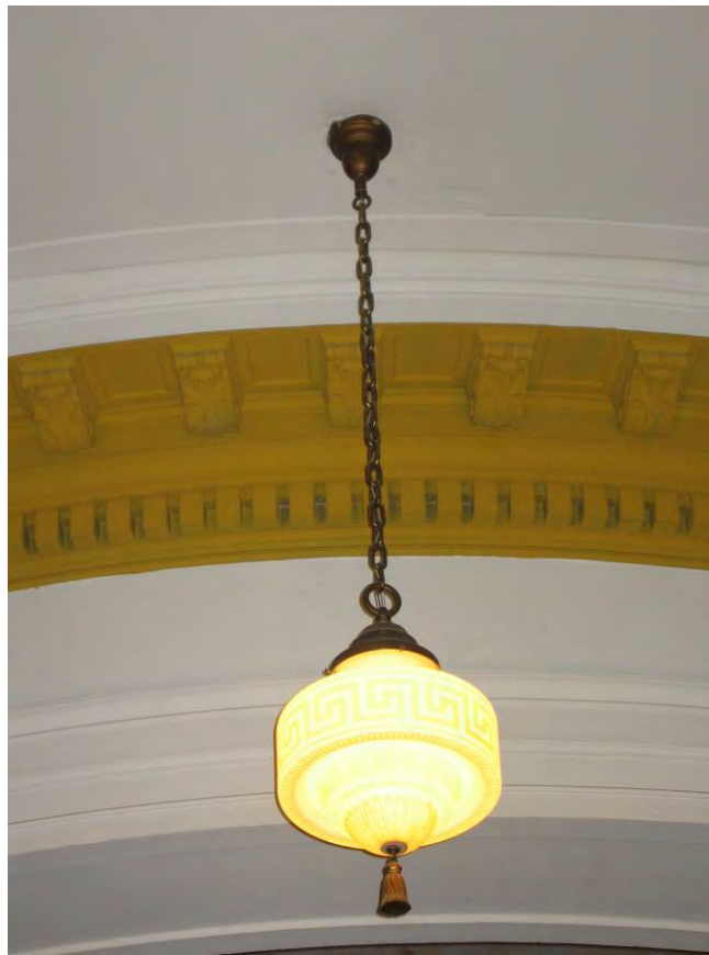
Example of original light fixture and cornice dentil and bracket moldings at the ceiling in the lobby
