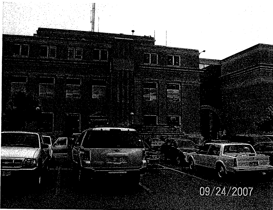
Pennington County Courthouse (South Façade)
