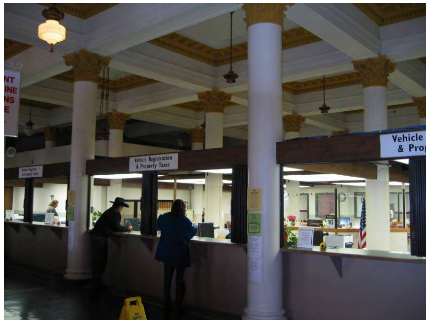
Second floor public counters; recessed ceilings with cornice details; columns with Corinthian capitals; original light fixtures
