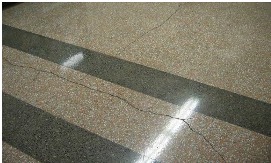
Third floor terrazzo floor cracks
