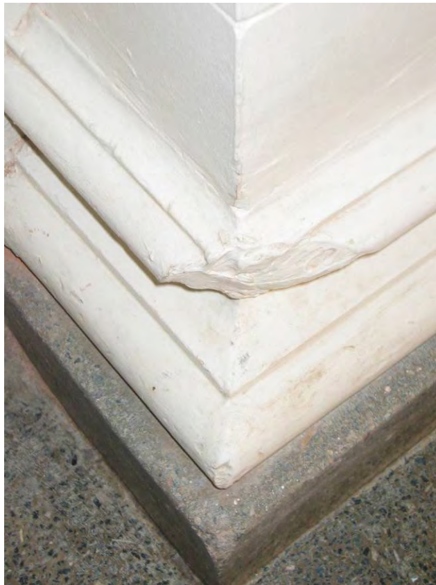
Example of chipped corner at base of pilaster on first floor
