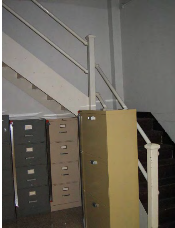
Stairs to west penthouse apartment
